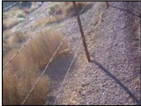
Standard 4-strand barbed wire fencing. Tortoise proof retro-fencing material is attached to this fencing.
